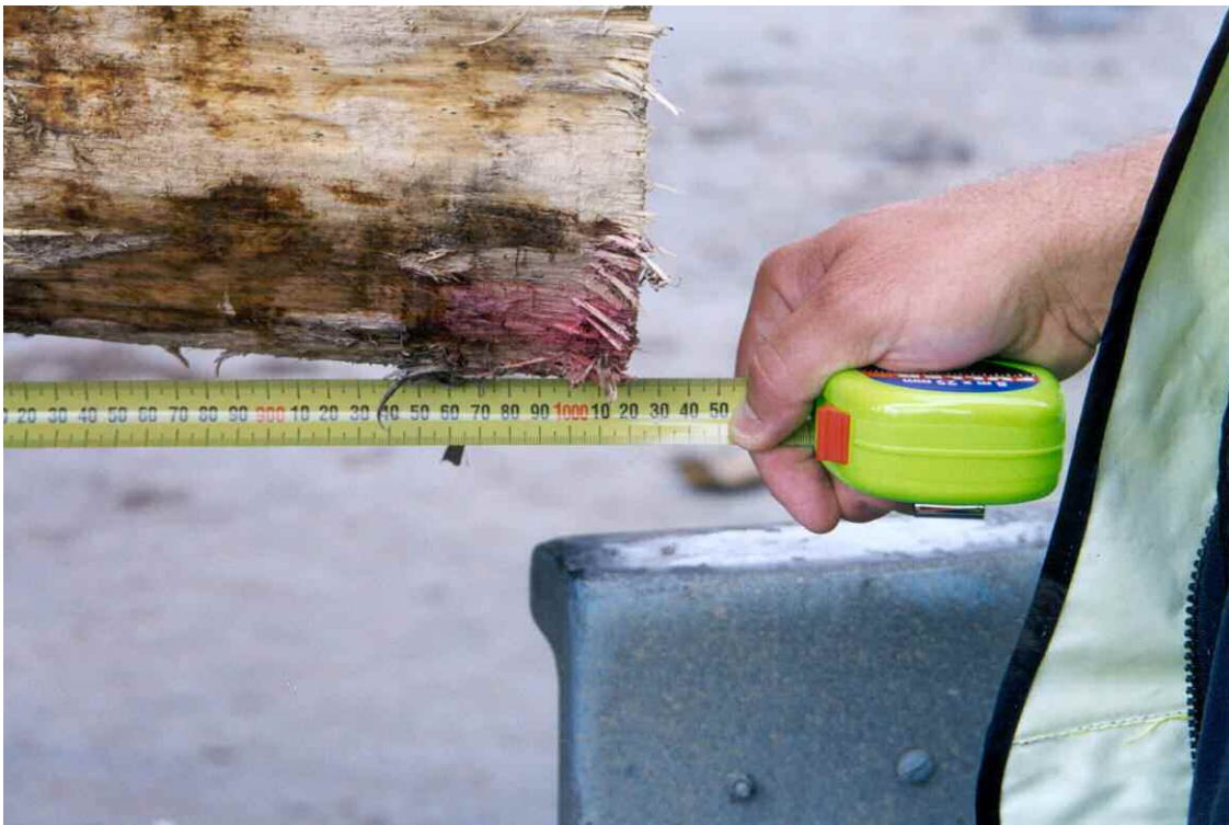
Photo 2 Minimum IVS (extent of front overhang of log beyond steelwork)
